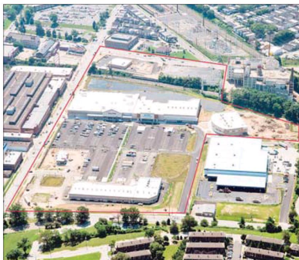
An aerial view of Bakers Centre in North Philadelphia, partly still under construction. The ShopRite opened Aug. 1.
